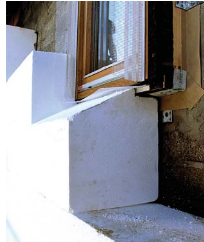
Externally insulated concrete block wall. Source: MosArt Architecture.
